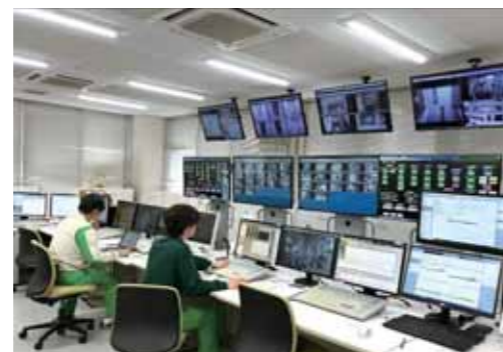
Smart factory in action at the Nagoya Plant
