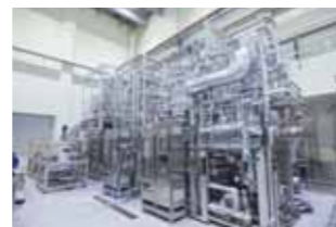
Some of the facilities for pilot-scale activities
