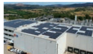
IQL (Spain) solar panels
