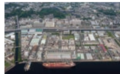
Yokohama Isogo Complex
